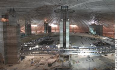
**Above:** The roof structure was built at ground level on a series of temporary trestles.
