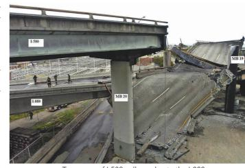
Two spans of I-580 collapsed onto the I-880 connector ramp directly below.
