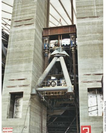
Each of the concrete cores at the eight points was designed so that the roof "slotted" into a gap in the core, allowing the roof to be lifted from directly above the bearing point.
