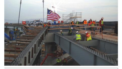
Built-up sections were fabricated with thicker web plates to minimize the number of stiffeners required. Flange plates were kept constant to simplify fabrication. The bridge reopend to traffic in only 25 days.
