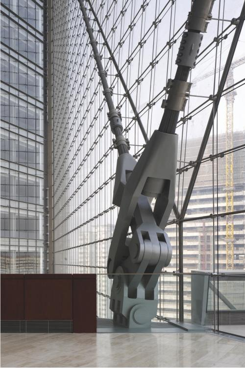
ing operations. The remaining boundary conditions were provided at the bottom of the net by the concrete structure at ground level, and at the top by a three-story-tall structural steel truss spanning 60 m (200 ft) between the top of the two cores.
